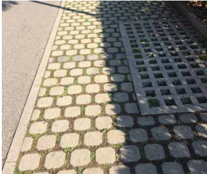
Figure 59: Examples of permeable paving (© Wikimedia Commons).
