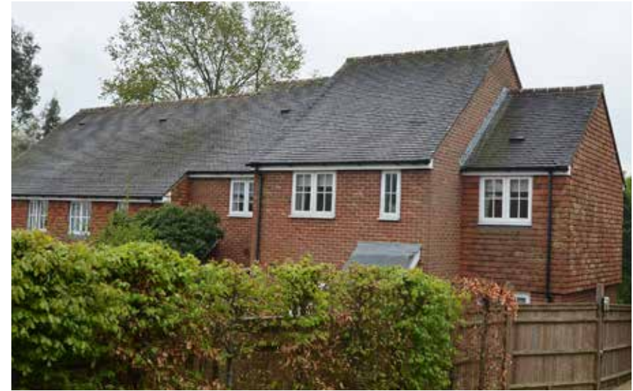
Figure 43: Contemporary development with variations in roof height and upper storey treatments that break the monotony of the row.
