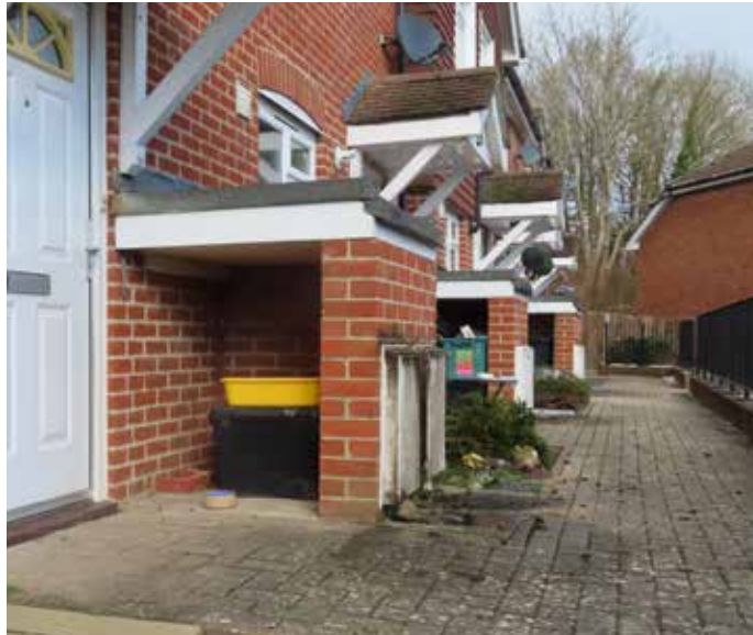
Figure 61: Bin stores made for waste boxes, now too small for “wheelie bins” © Bev Marks 2021.
