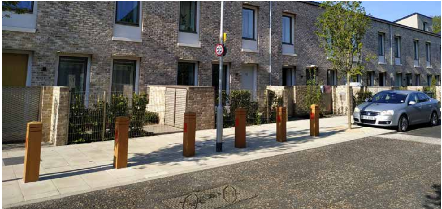
Figure 20: Example of a raised mid-block pedestrian crossing on a 20 mph street on Goldsmith Street, Norwich (note: many local authorities require blister tactile pavers at crossings to guide visually impaired pedestrians).
