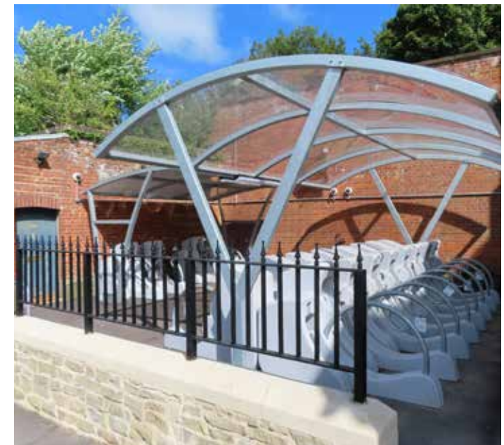
Figure 35: New roofed cycle rack with rail indicator screen and CCTV at Battle Station ©Bev Marks, 2019.
