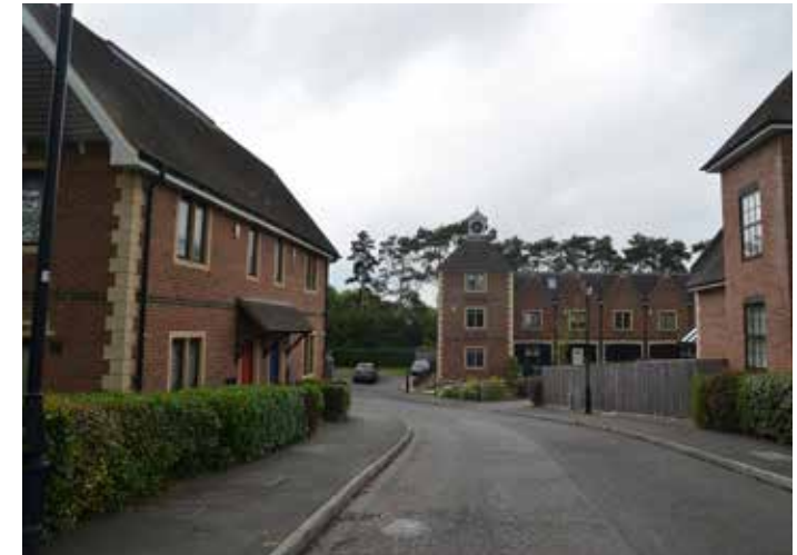
Figure 16: Contemporary residential buildings on Sunny Rise arranged in small clusters and terraces around mews and courtyards.
