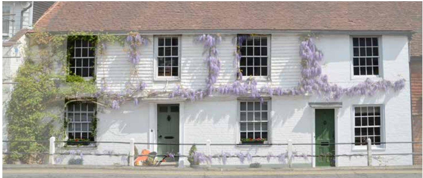
Figure 49: Building displaying a consistent traditional window style and shape across the main elevation.
