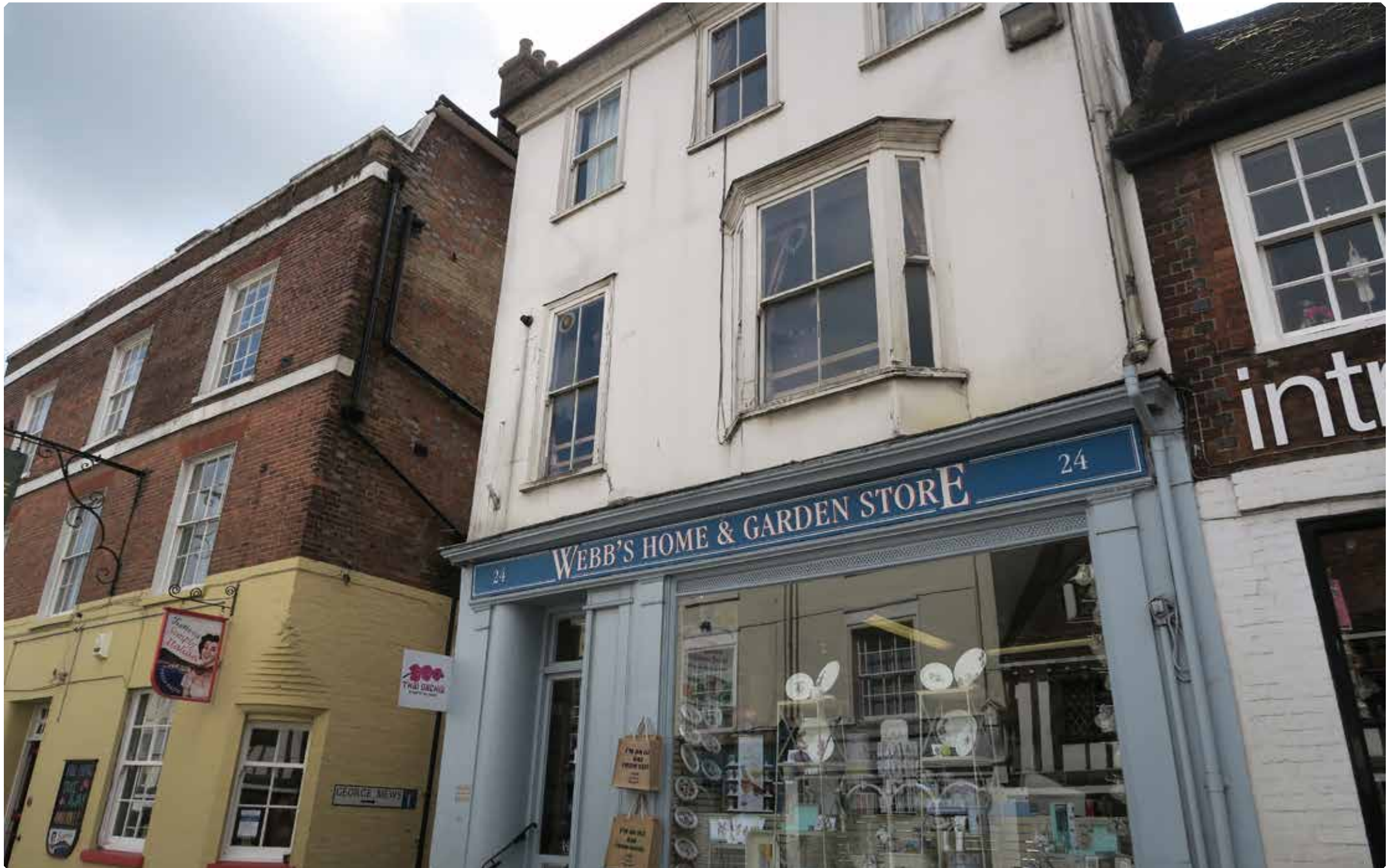
Figure 75: High Street shopfronts and listed buildings.
