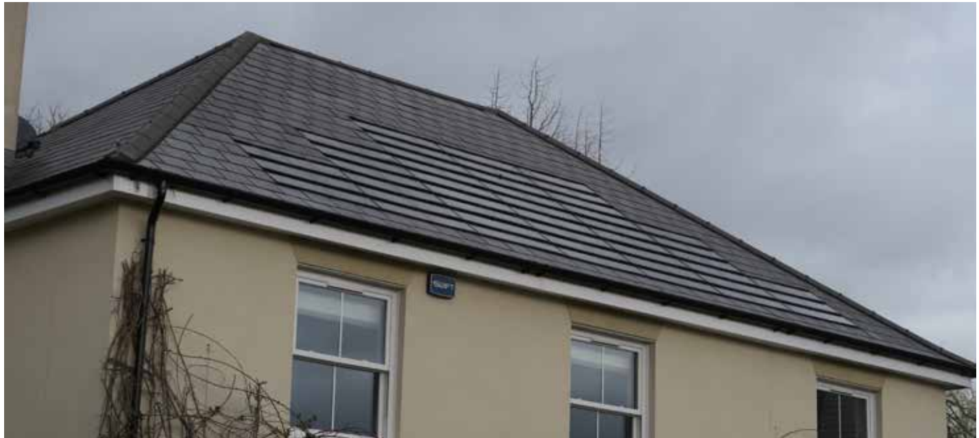
Figure 65: Use of low-profile solar shingles on a slate roof in Lingfield, Surrey. The shingles are laid flush with the surface of the roof and integrated into the roof system. Note: photo for illustrative purpose only; the use of slate is not recommended in Battle Civil Parish.
