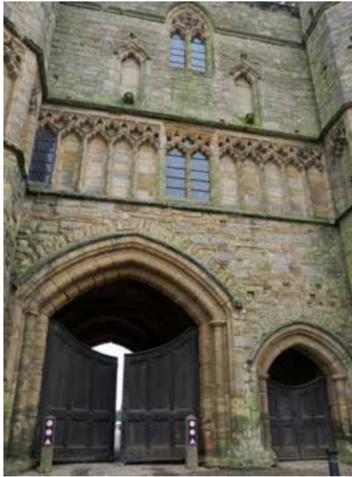
Battle Abbey Gatehouse - Gothic pointed carriage archway and ornamental first floor arcading.
