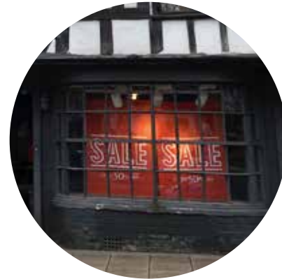
Multi-pane shopfront display window
