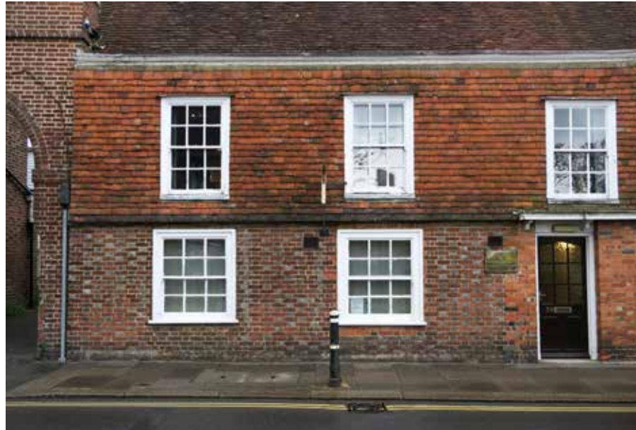
Figure 48: House displaying consistent window colour and styles.
