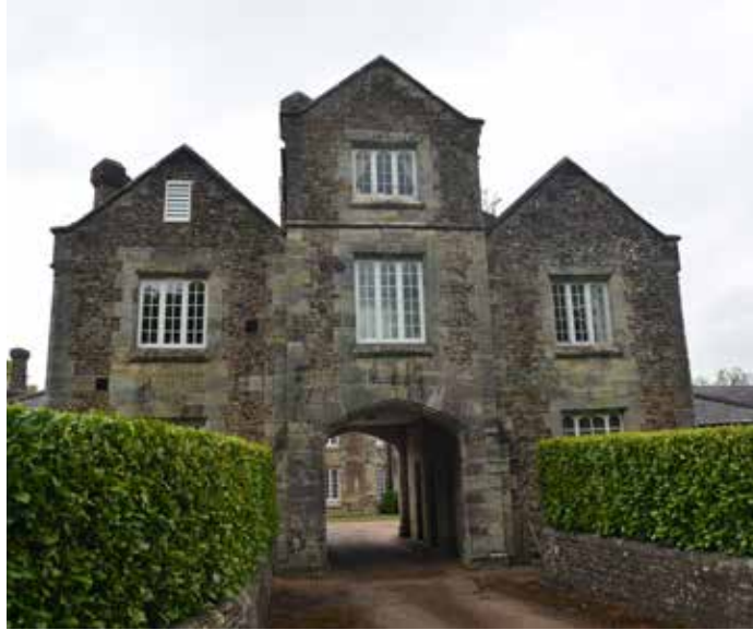
Figure 45: Battle Hospital Gatehouse flanked by hedgerows and low walls.
