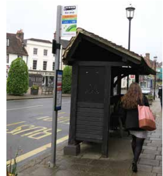
Figure 53: Bus shelter built with traditional local materials.
