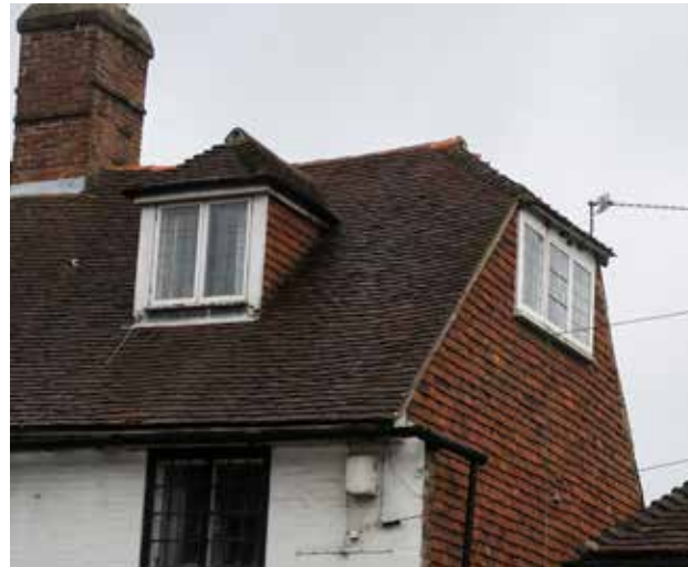
Half hip clay plaintile roof, hipped dormer, white painted façade, and gable clad with hung clay tiles.
