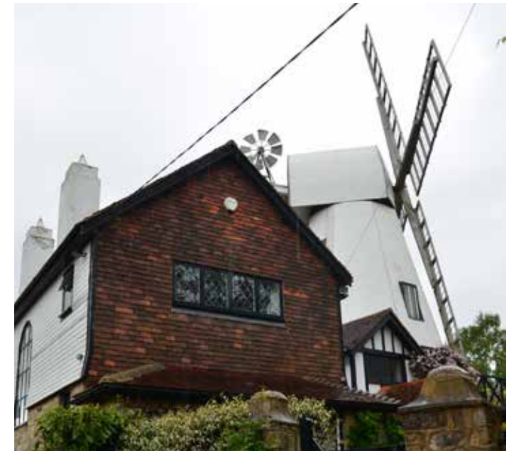
Figure 8: Grade II listed windmill on Caldbeck Hill.
