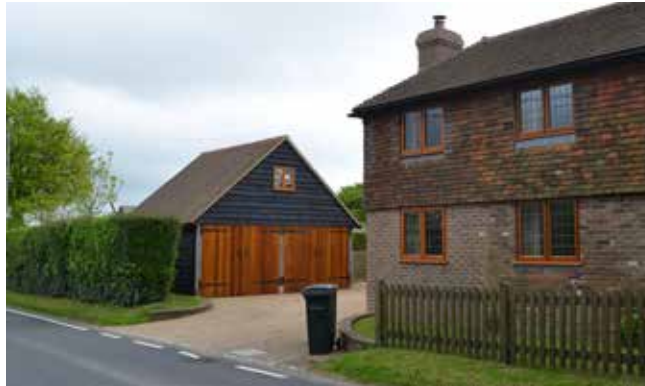
Figure 28: New garage built with local traditional materials.
