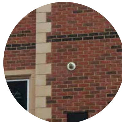
Red brick infill with sandstone trim
