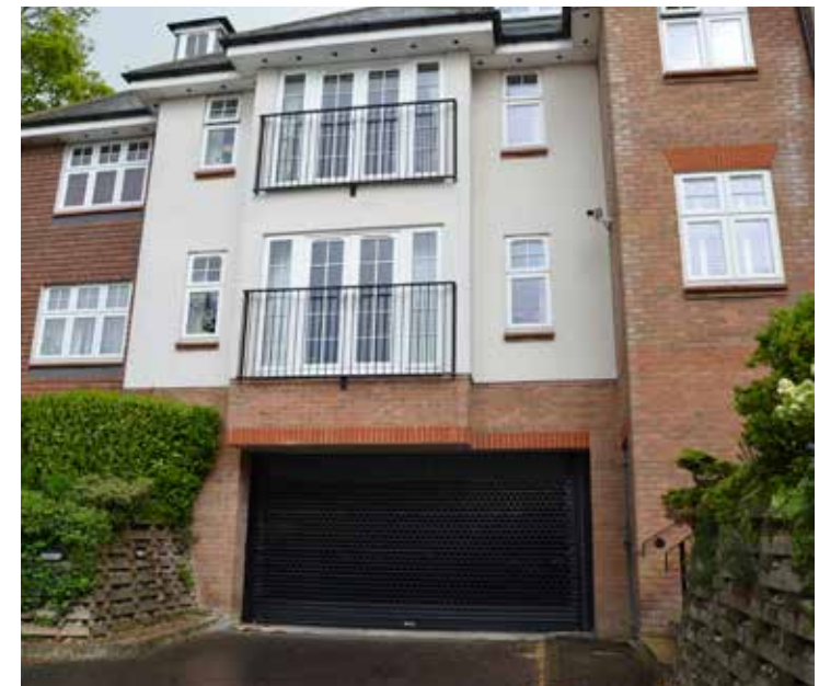
Figure 32: Apartment building with undercroft parking entrance partly screened with landscaping.
