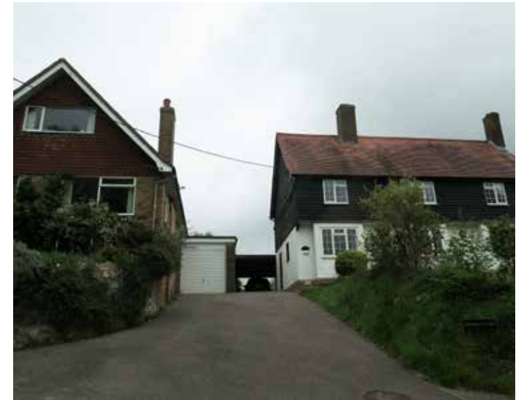
Figure 31: Single-family houses with side garages set back from the main building line.
