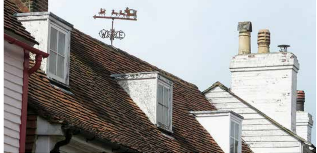
Clay plaintile roof with shed dormers and decorated weather vane.
