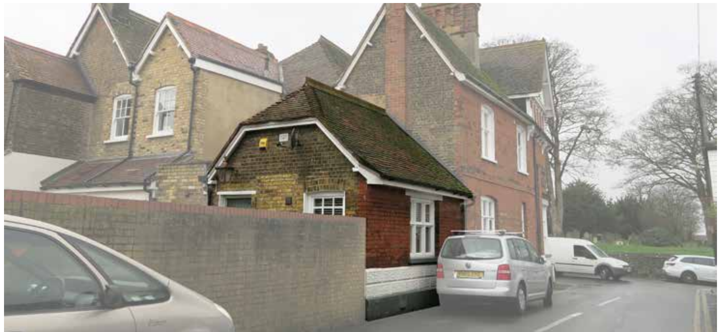
Figure 50: Examples of positive designs for side and rear extensions in Cliffe, Kent.
